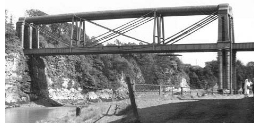
a. Guenzburg bridge, Pauli, 1853 (Culmann 1866) b. River Wye bridge, Brunel, 1852 Figure 6. Structural forms deviated from experience and scientific investigations.
