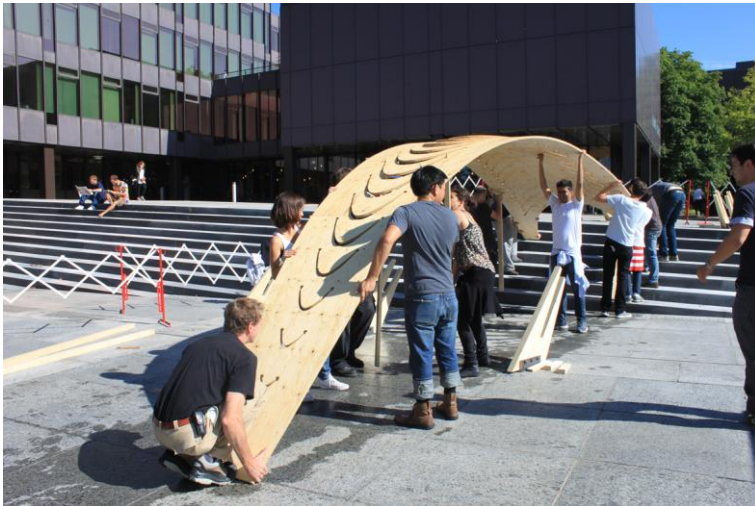
Figure 8. Manually bending the central plywood panel during the construction phase.
