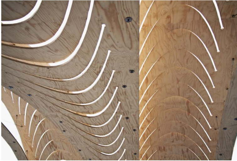
Figure 3. Detail of the lamellas working as sun louvers integrated into the design. The cuts allows for the curvature of the bent panels to be adjusted.
