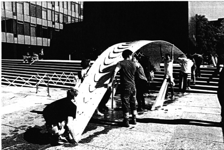
Fig 16. ETH/AA-Pavilion Simple construction of pavilion through bending
