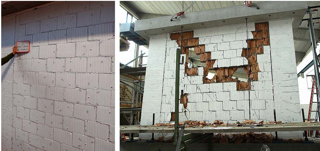
Figure 10. Failure patterns of specimens S1 and S2.
