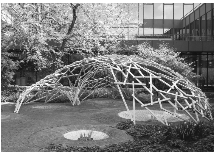
Fig. 1: Two examples of Reciprocal Frame Structures (left [6]; right [5])
